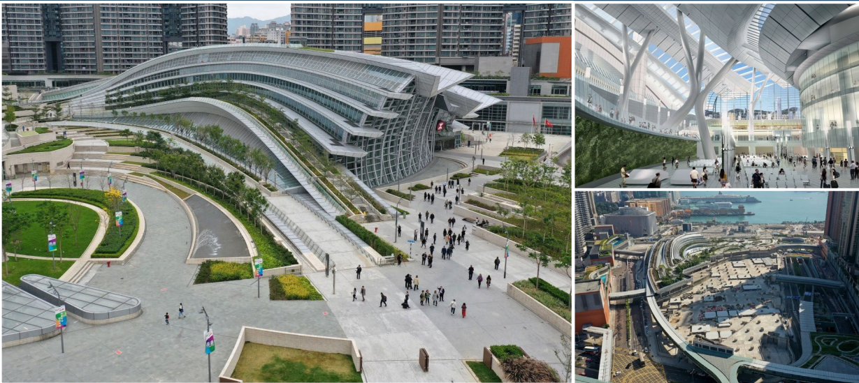
Hong Kong HSR West Kowloon Station
