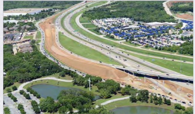
April 2015 -- SH121/360 ramp progress
