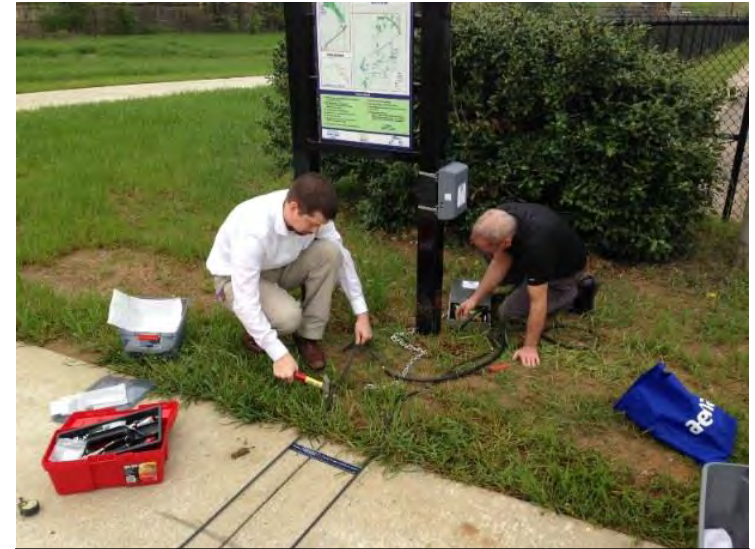
Installation of a mobile counter on the John Barfield Trail in North Richlands Hills
