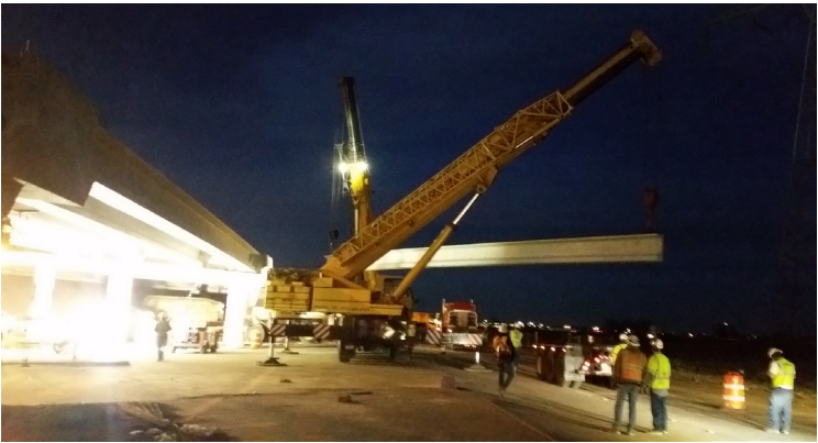
Beam setting on Thoroughfare B, the U-Turn Lane South of the Spring Creek Parkway.
