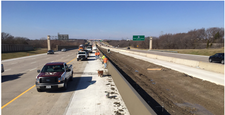
Newly constructed concrete traffic barrier for PGBT fourth lane.
