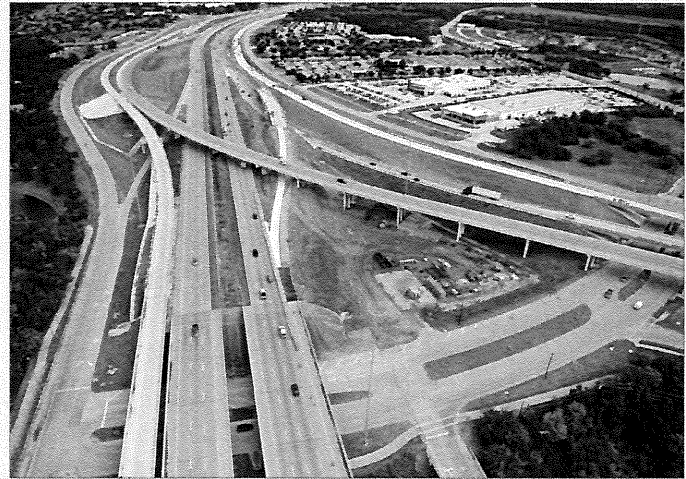
SH 121/360 interchange construction
