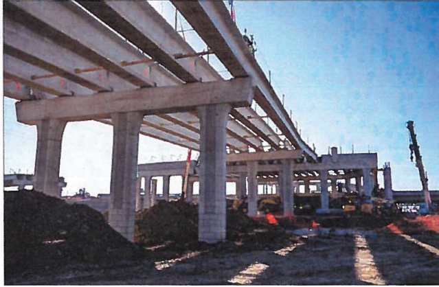
Above: Precast beams for direct connector bridge at SH 183
