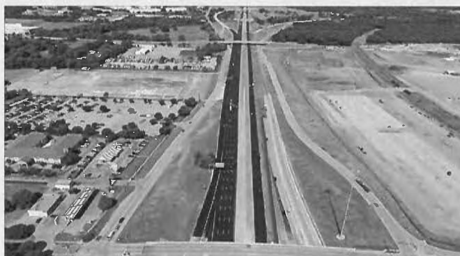
MAY 2018: Final paving and striping on SH 183 west of SH 161
